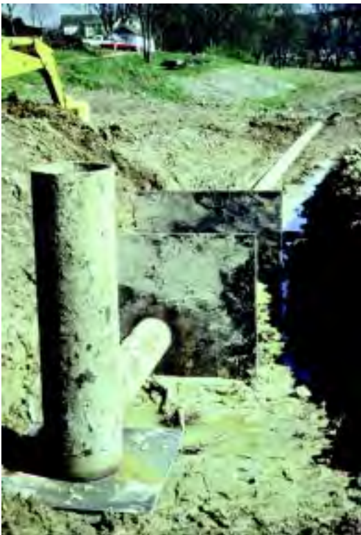
Figure 22 Drop-inlet pipe spillway with antiseep collar
