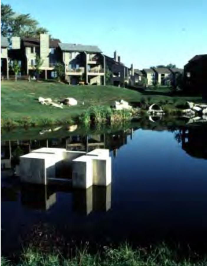
Figure 10 This pond, which served as a sediment basin while homes in the background were being constructed, now adds variety and value to the community
